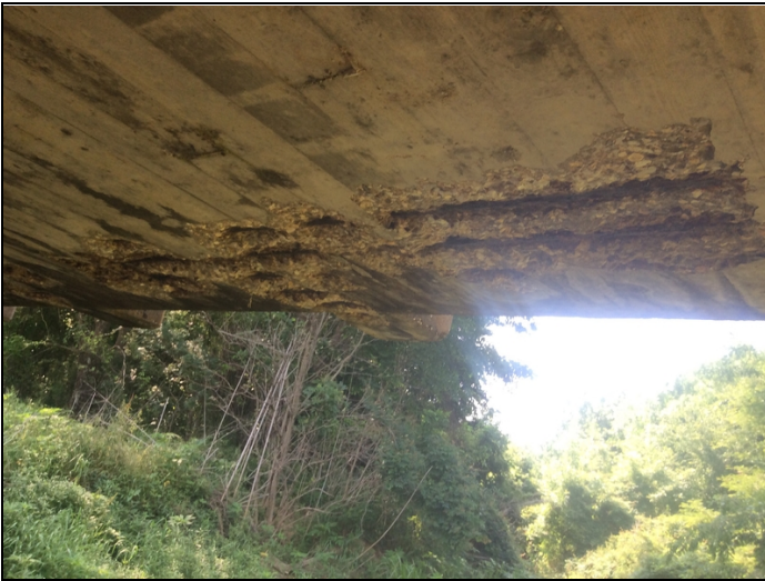
Spalls with exposed rebar at span 1 right side of soffit area near midspan towards bent 2 .
