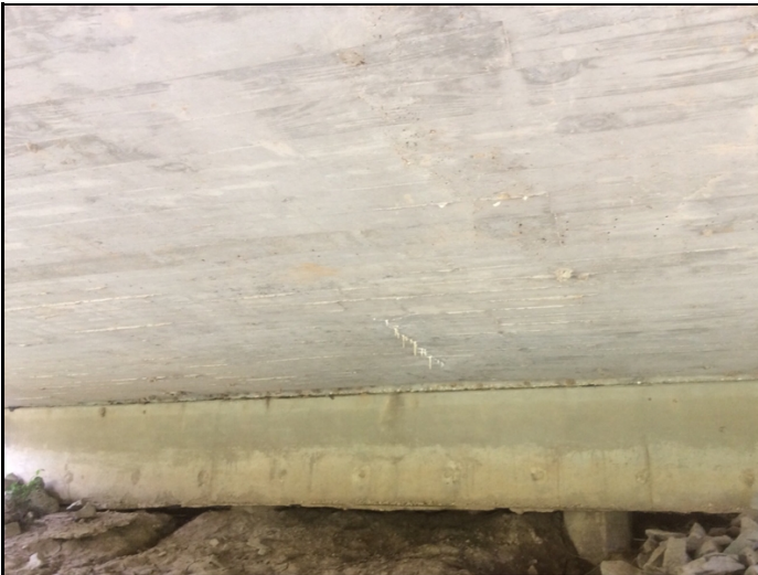
Soffit - Span 2 @ Bent 3 (efflorescence)
