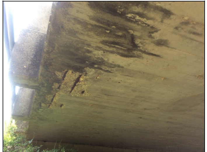
Soffit - Span 2 left (rebar exposed)
