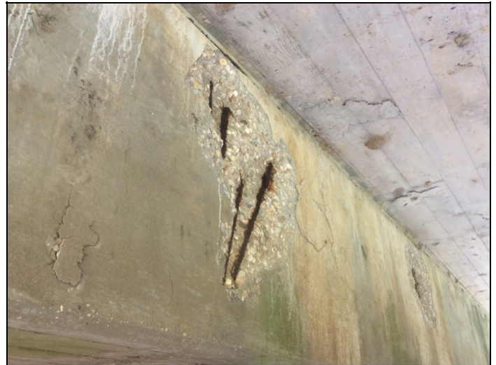
Cap - Bent 2 back (rebar exposed)
