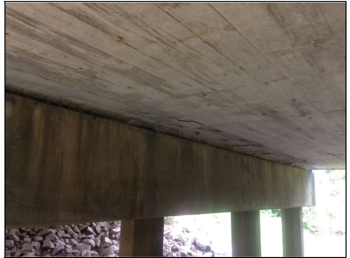
Soffit - Span 2 @ Bent 2 (delaminations)
