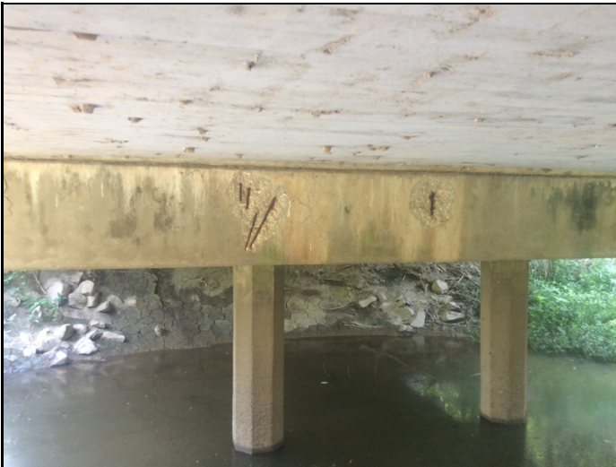
Bent 2 cap back has spalls with exposed rebar.
